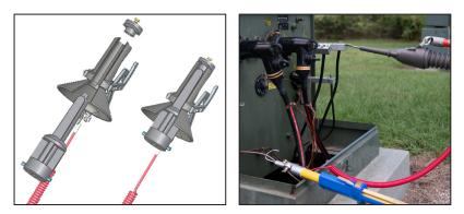
\*Using the Auto Clamp Adaptor is not required if the end of the Extension Cable can securely clamp to a bare grounded cable.
